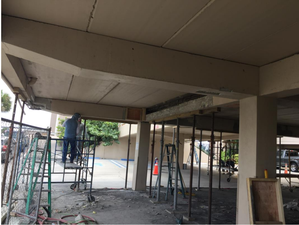
Picture 3: In-progress demolition
