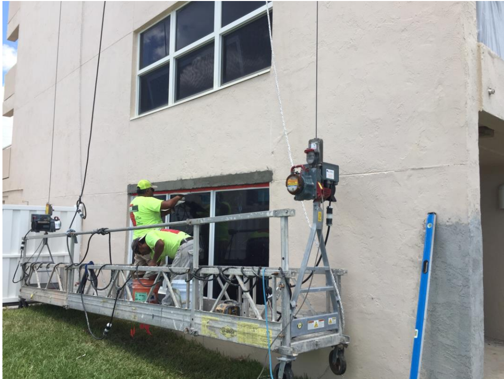
Picture 4: In-progress stucco application
