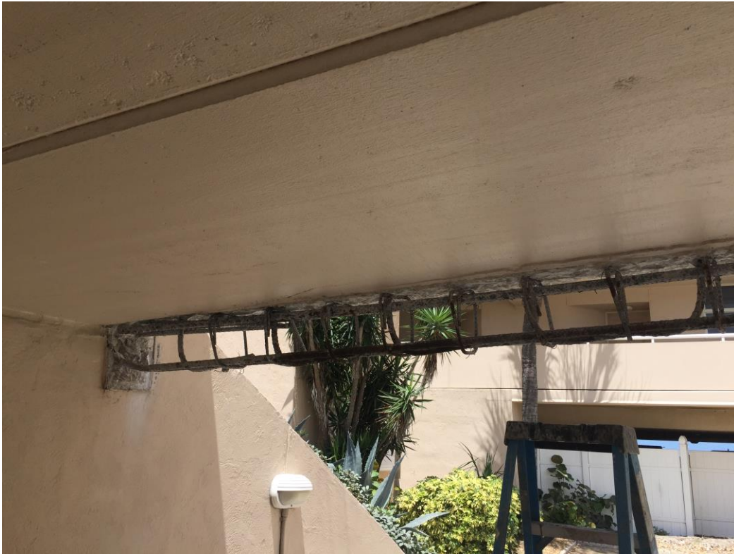
Picture 1: Completed excavation prior to sandblasting
