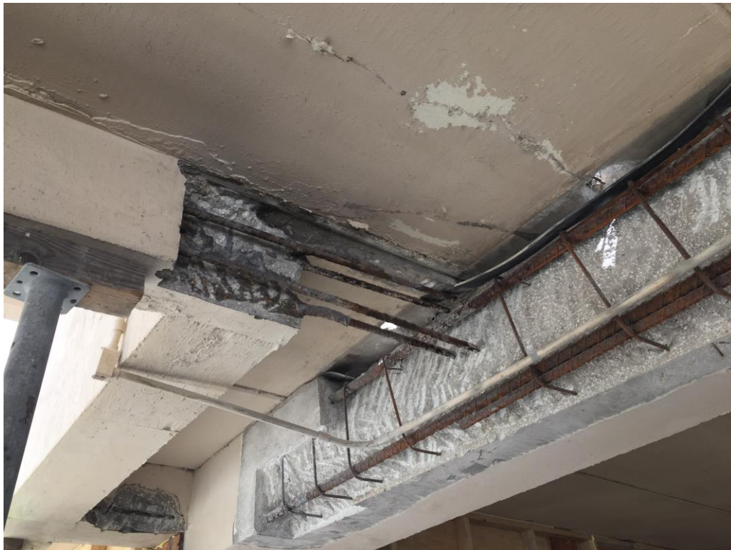
Picture 2: Completed excavation prior to sandblasting
